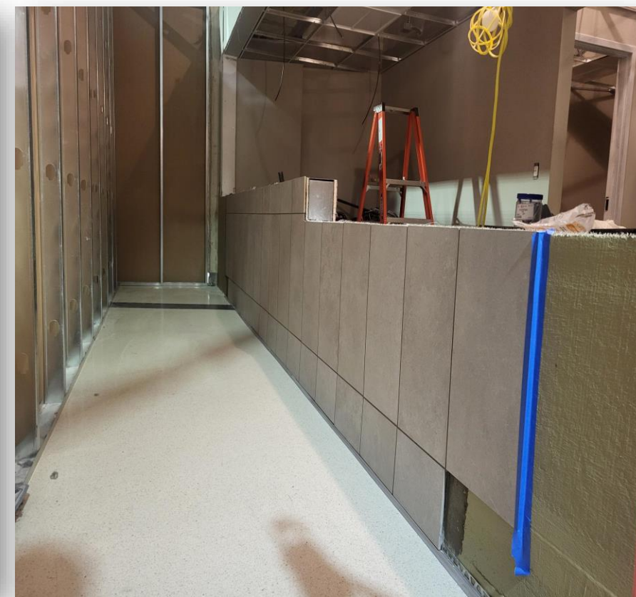
Revenue Counter New Tile Installation
